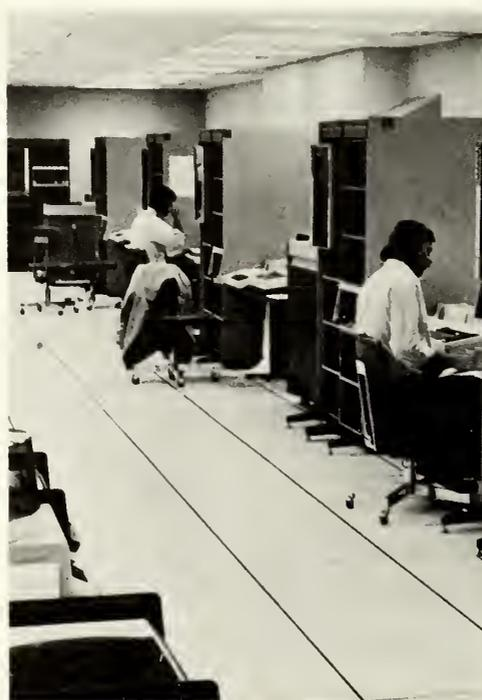
Computers such as these (enclosed in cabinets on the righthand wall) are the nerve centers of the GPO photocomposition system. The computer on the rear wall can perform page make-up.
