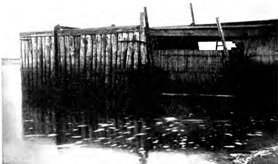
Fig. No. 9.—Side View of the end of the Hatchery Wharf showing the latticed pens for mating and berried lobsters and admitting a tidal flow of water. Near the end of the wharf may be seen the intake pipe which supplies sea-water to the hatchery jars and rearing boxes.
