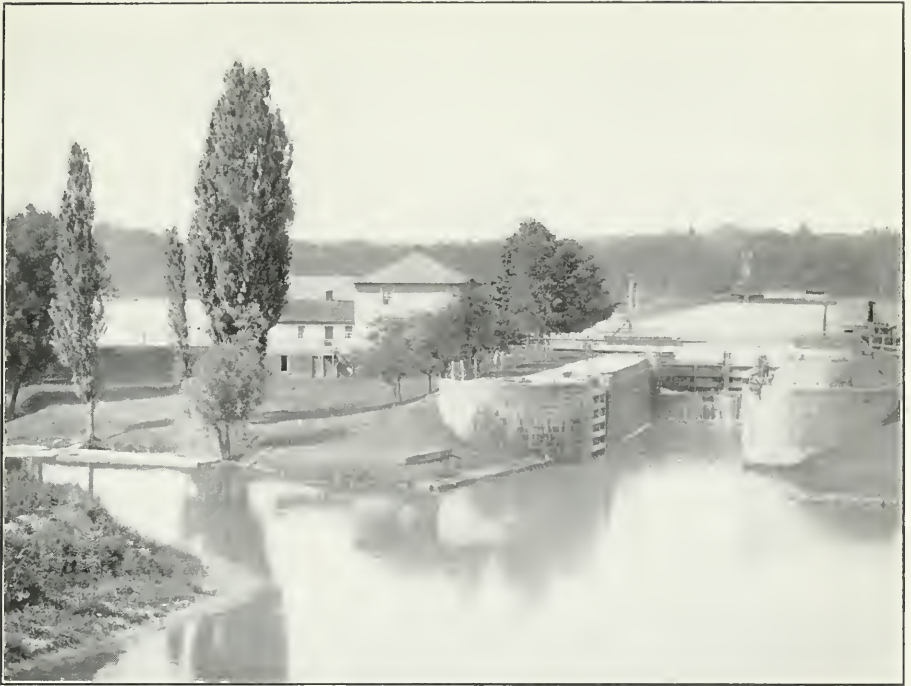
Rideau Canal. Washburn Lock.
