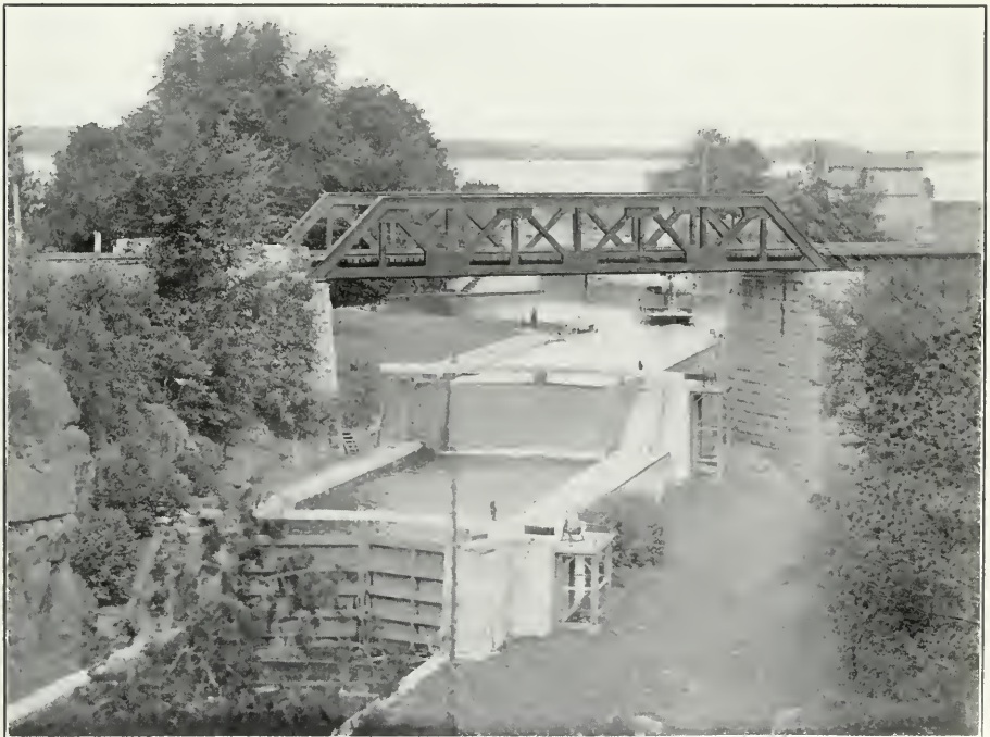
Rideau Canal. Kingston Mills, with Grand Trunk Railway main line overhead crossing.
