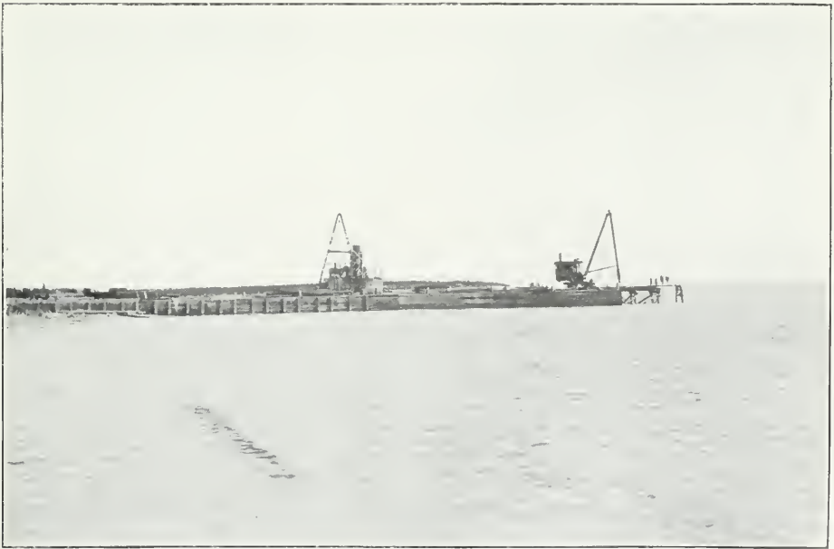
Hudson Bay Railway. Wharf No. 3, Port Nelson.
