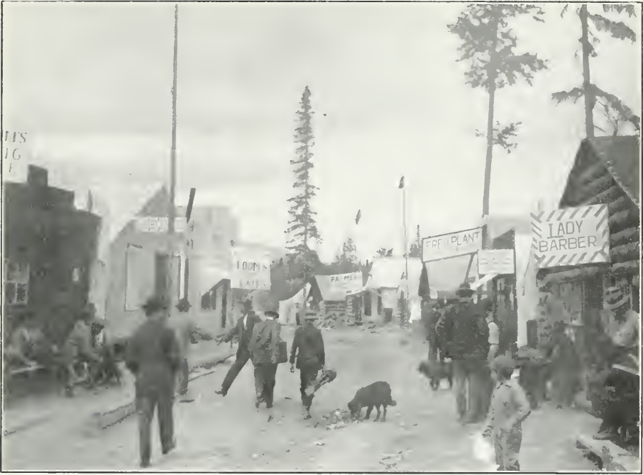
Grand Trunk Pacific Railway. Tête Jaune Cache, during the construction of the railway.
