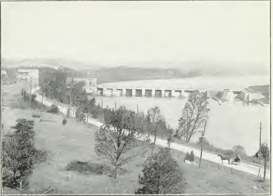
Trent Canal. Lock and Dam No. 2, at Trenton.
