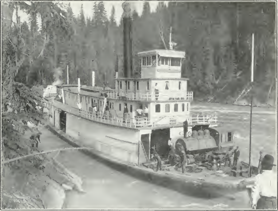
Grand Trunk Pacific Railway. Transporting contractors' supplies down the Fraser river, B.C.
