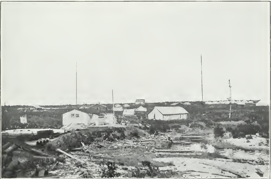
Hudson Bay Railway. Eastern end of encampment, showing wireless installation in background.
