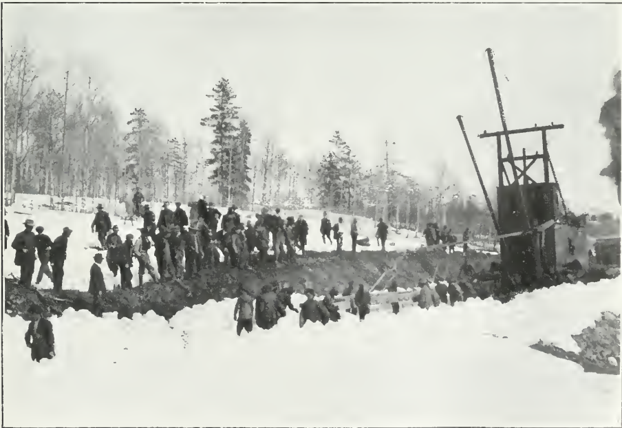
Grand Trunk Pacific Railway. Laying the last rails, Central British Columbia.
