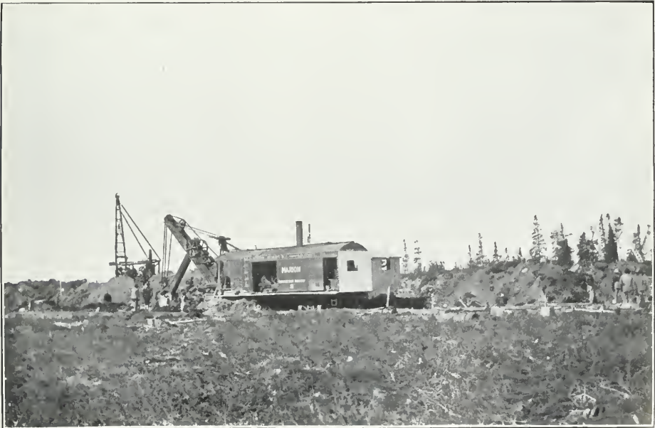
Hudson Bay Railway. Steam shovel at work, Port Nelson.
