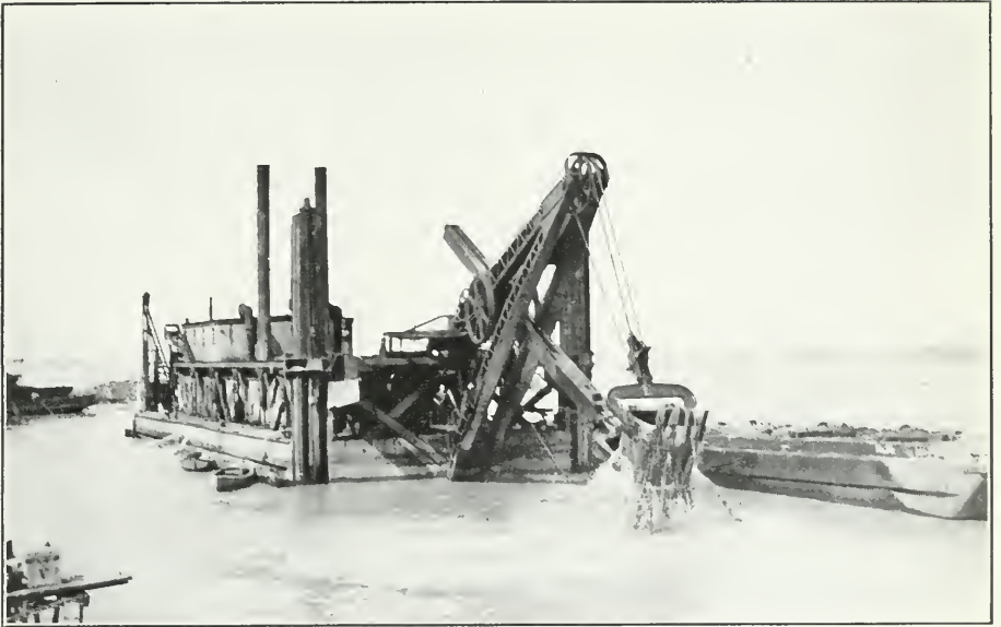
New Welland Ship Canal. One of the large dredges at work at Port Weller, Lake Ontario.
