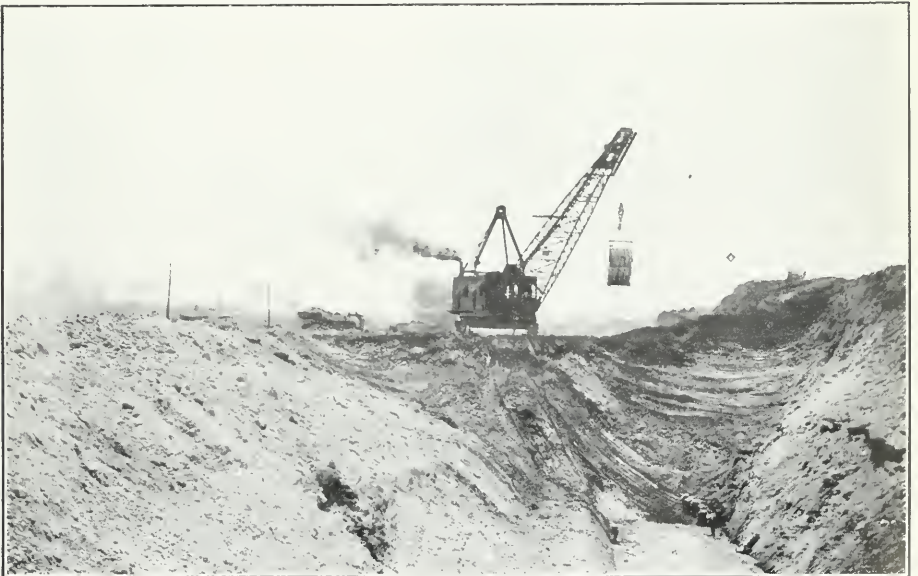
New Welland Ship Canal. Trench for entrance wall, Lock No. 1.
