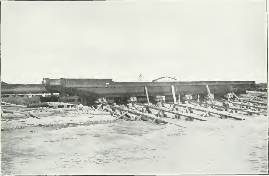
Hudson Bay Railway. Hull of stern wheel tug assembled and ready for launching.
